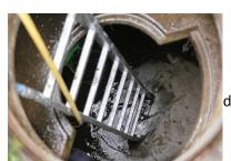
Any liquids should be pumped out of a confined space and liquid flow diverted from the space before testing for toxic gases is carried out. If the liquid cannot be removed then it should be stirred as vigorously as possible while testing takes place. The stirring should be mechanical using a stirrer or pump, or by blowing compressed air through the bottom of the space.
