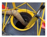
You need to be careful that people outside the confined space are not exposed to gas while the atmosphere inside the confined space is being purged. You also need to be careful when purging flammable gases.
