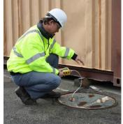
You need to make sure any torches or communication equipment is safe to use in a confined space.
